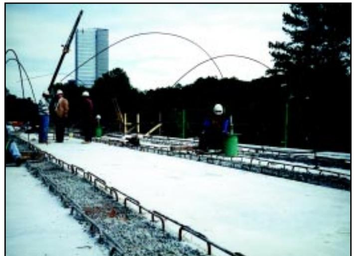
These construction crews use Simplex Hard-Kor™ hollow cylinders to pre-tension steel rods in cast concrete forms. "The Hard-Kor™ cylinders, with their leak-proof base and extra power, made a tough job easy."
