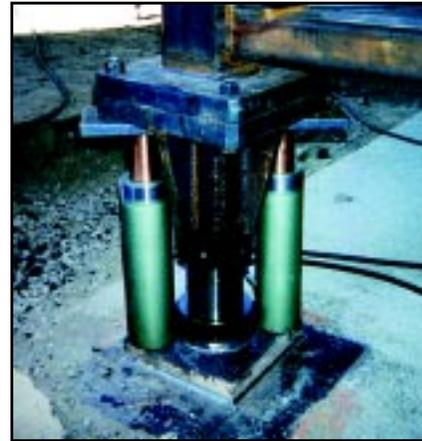
Contractors called on the brute force of Simplex R5513 cylinders to lift and position highway ramps in San Diego. PE50 power units provided the power and control in this rough outdoor application.
